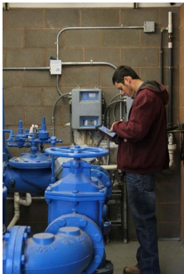
Figure 2. On-site measurements of flow, head, and power enable calculations of wire-to-water efficiency.
