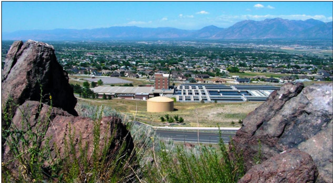
Jordan Valley Water Treatment Plant in Herriman (view is from the southwest near Mountain View Corridor looking northeast)
