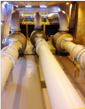
Jordan Aqueduct Reach 4 Near Point of the Mountain
